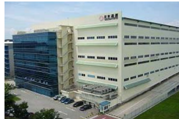
Hi-Speed Logistics Centre
